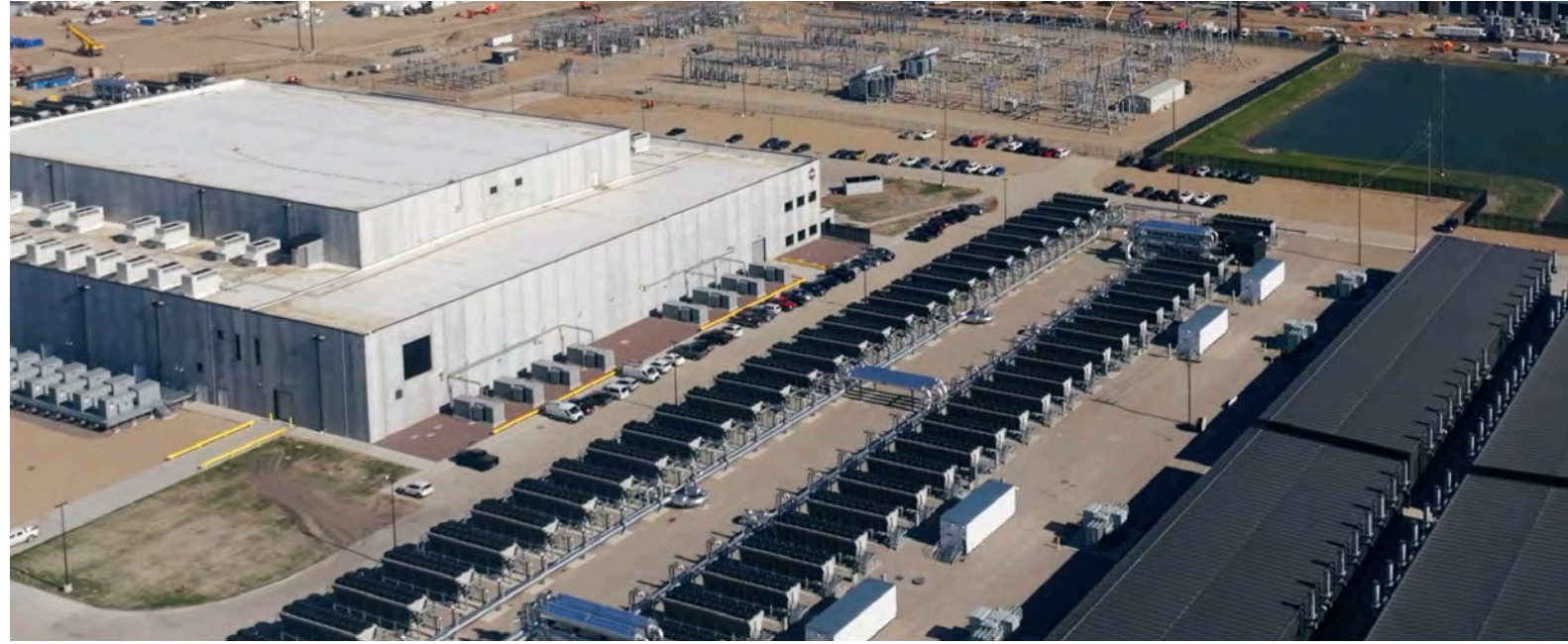
Building 1 - 100 MW - Pilot Build (PF1-1)
