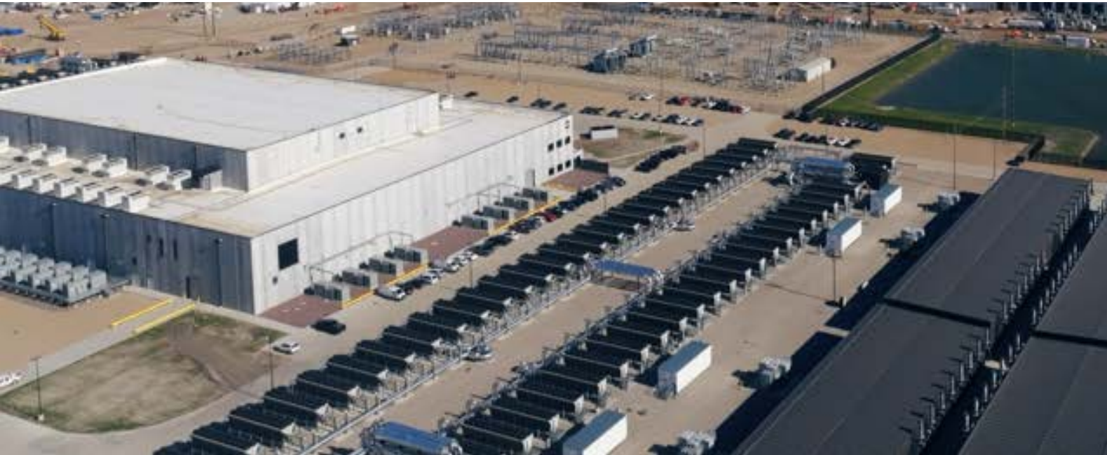
Building 1 - 100 MW - Pilot Build (PF1-1)
